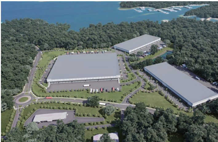
Metro Atlanta Industrial Development Project (Georgia, U.S.A. / Expected Completion: 2026)
